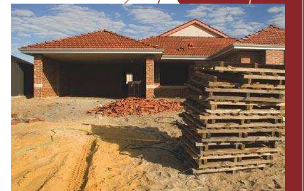
Basic initial waste management practices On-site sorting of "heavy" waste allows these materials to then be recycled cost-effectively. These basic initial waste management practices will become more sophisticated as Smart Builders evolves.
