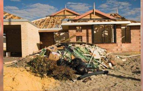
What Smart Builders is trying to change Standard existing practice for construction sites on large residential developments is a pile of unsorted mixed waste – the vast majority of which goes to landfill.
